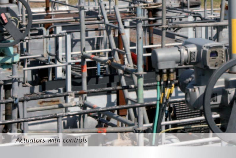
Actuator controls with integral local controls are available for the actuators SA up to size 16.2 and all part-turn actuators SG. They form the optimal interface between process control and actuator.
