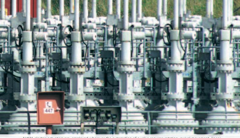
AUMA electric actuators are employed wherever the automation of a valve requires rotation, swivel movement, linear movement or actuation via a lever.
